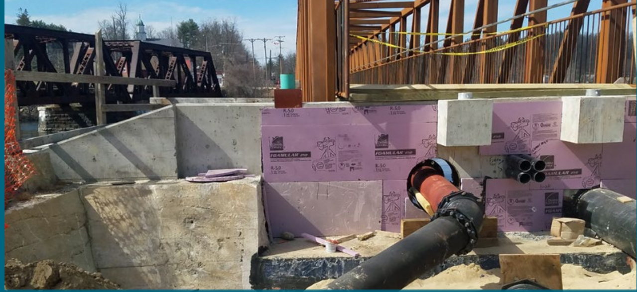
Utilities are replaced without service interruptions.
