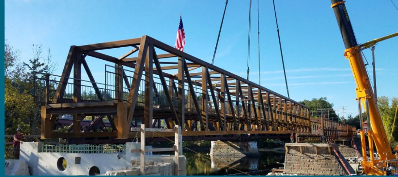
38-second time lapse bridge installation video: youtu.be/p1Ds0ZE2UQg
