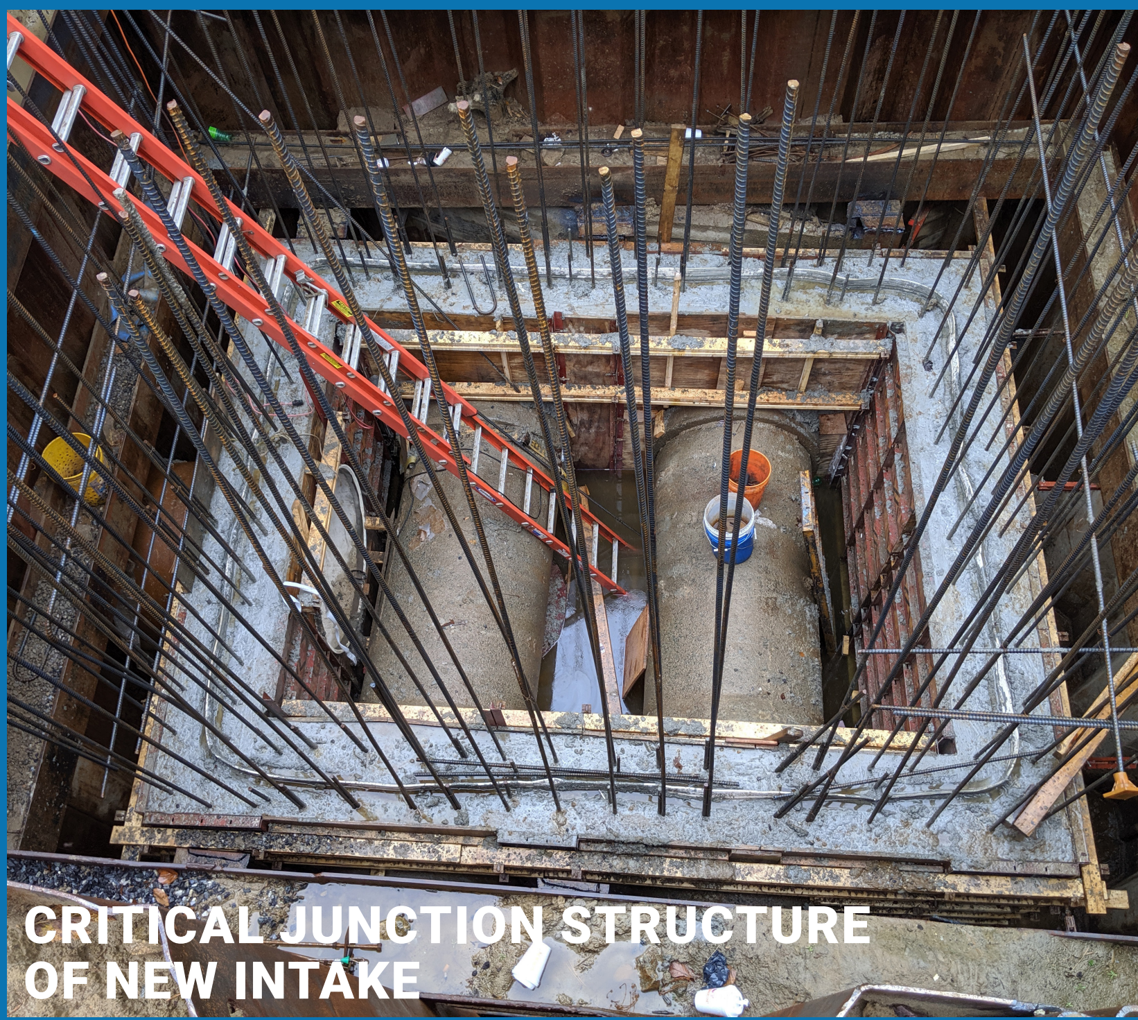
THE PIPE CROSSING READY TO BE SET IN PLACE AFTER 15 HOURS OF STAGING
