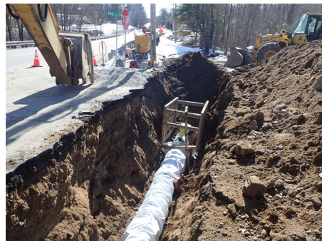
Typical Installation of 20-Inch Water Main
