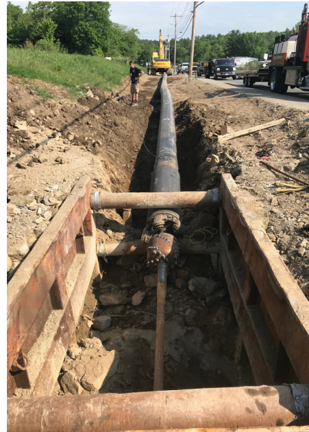
HDD Pipe Pull Back
