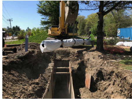
16-Inch Open Cut Crossing of Range Road
