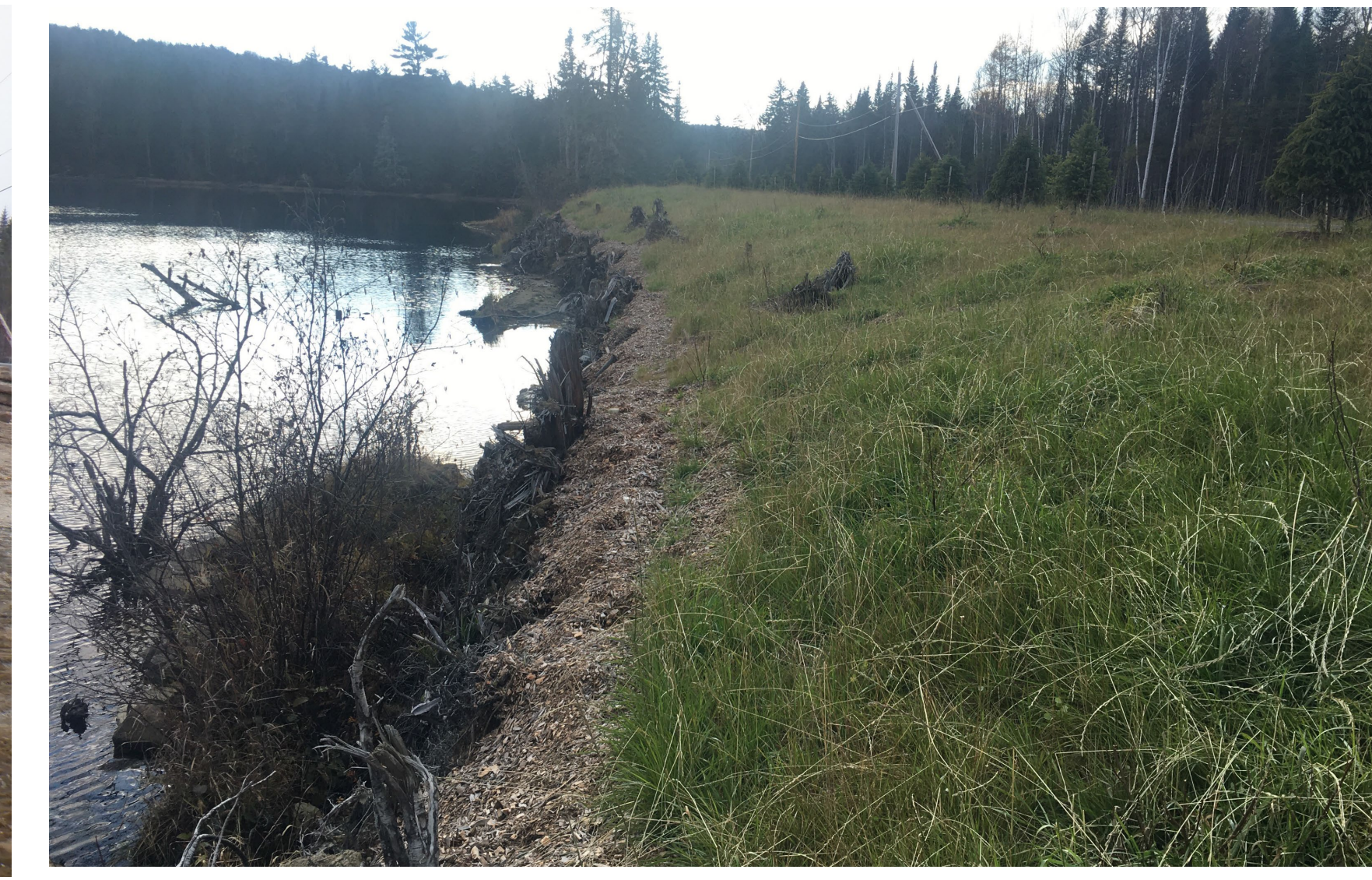
Post-Construction 11/8/2021 The Completed Project: With stable root fans and plants growing. The project was uniquely developed and constructed with close coordination between the owner and roadway designer (NHDOT), designer and construction oversight of the bank stabilization project (SLR); member of the bank stabilization team (MJ); and the contractor (J.P. Sicard).
