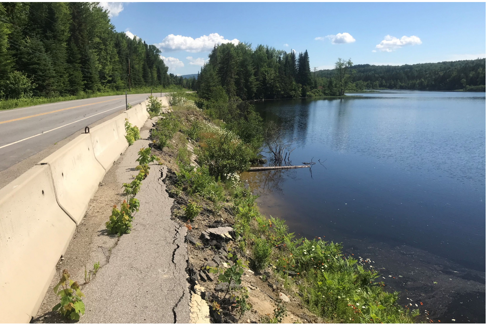
Pre-Construction 6/26/2020 Photo illustrates bank erosion and failed roadway prior to the project. The Challenge: Difficult and costly to stabilize the riverbank and accommodate and treat stormwater runoff with the road's current location in the environmentally sensitive Umbagog National Wildlife Refuge.
