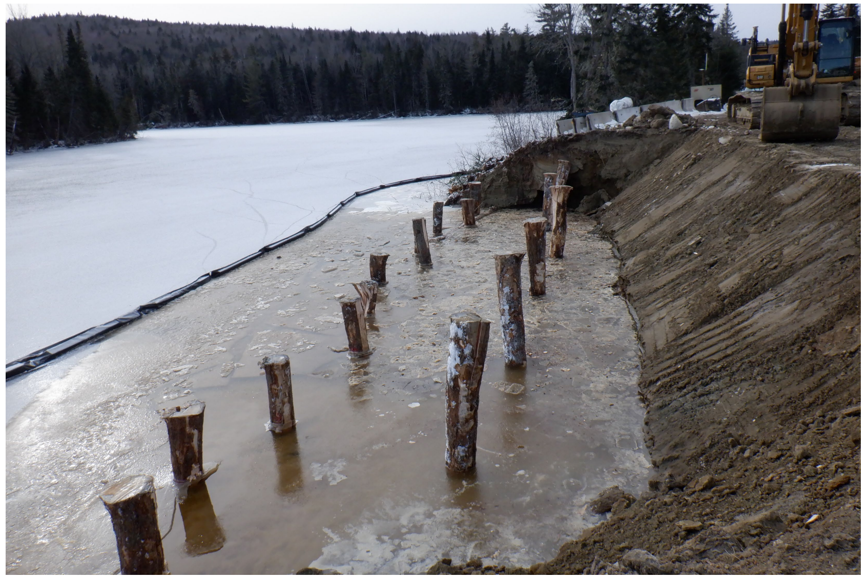
Construction 12/18/2020 The Engineered Solution: A Cost-Effective, Self-Sustaining, Resilient Design in an extremely Environmentally Sensitive Area. Photo shows placing of the initial key logs between piles.
