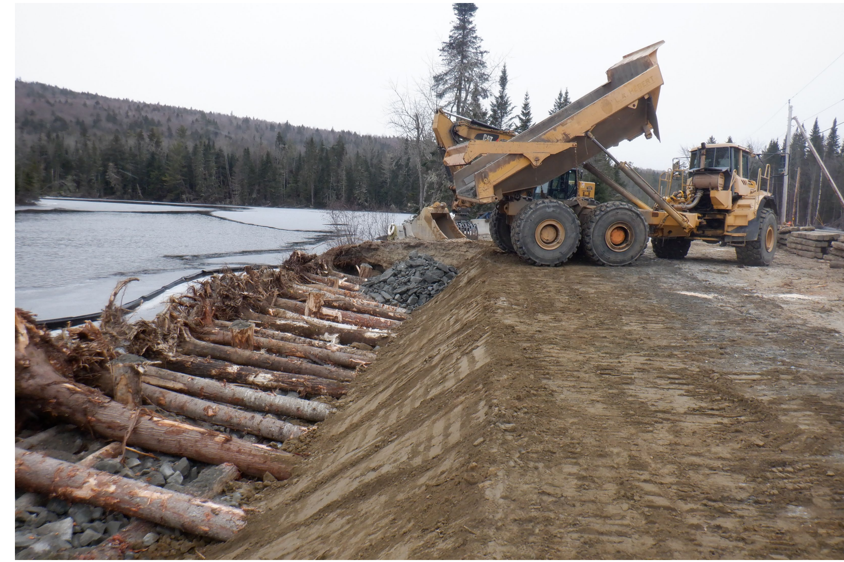
Construction 12/28/2020 Photo shows the Installation of stacked logs over the ballast. The project provided value to the engineering profession by providing a successful installation of the Ballasted Tree Revetment approach in New Hampshire, to use as a guide for future applications.
