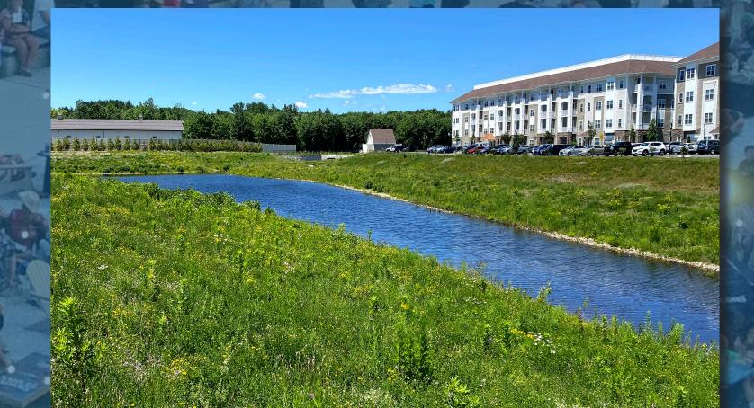
The finished daylighting of Policy Brook created more than 3,000 linear feet of natural stream and adjacent floodplain.
