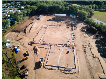
Building foundations in place, and sub-slab utilities being installed
