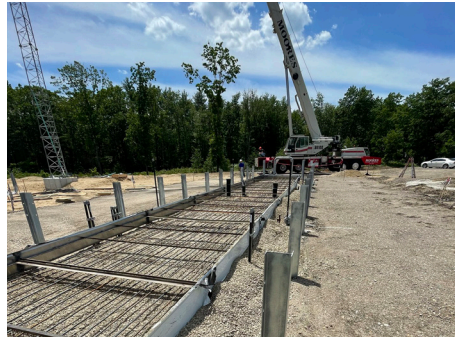
New concrete pad for above ground fuel tanks under construction
