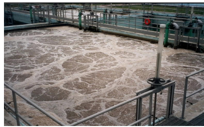
Plug-Flow BNR Reactor
