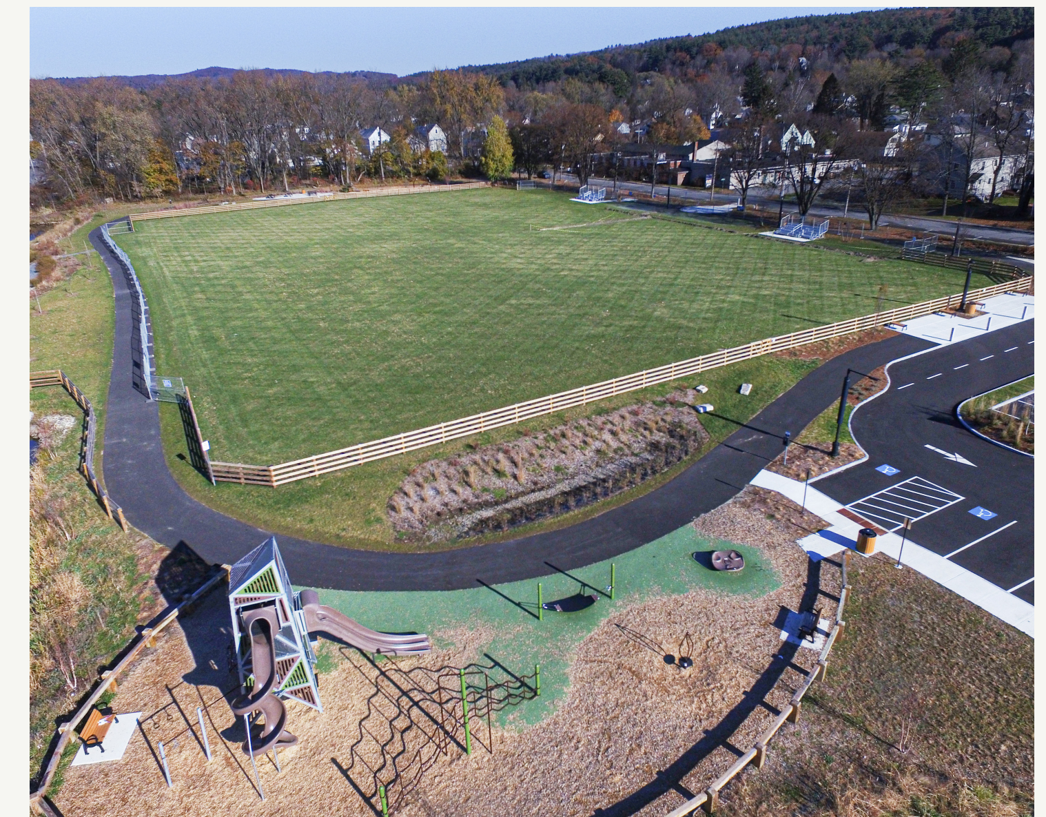
Post-construction aerial showing completed field; new stormwater basin/wetland; new bank stabilization along Beaver Brook; Solar lighting; improved access, circulation and parking.
