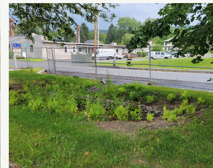
One of many rain gardens which were incorporated into the design to collect and treat runoff water from Carpenter Street.
