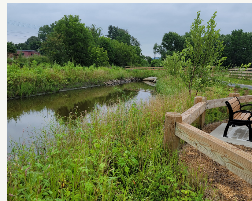
A replaced properly sized pipe diverted stormwater from Carpenter Street to this new storage basin/wetland system, which also serves to treat the water prior to discharging to Beaver Brook.
