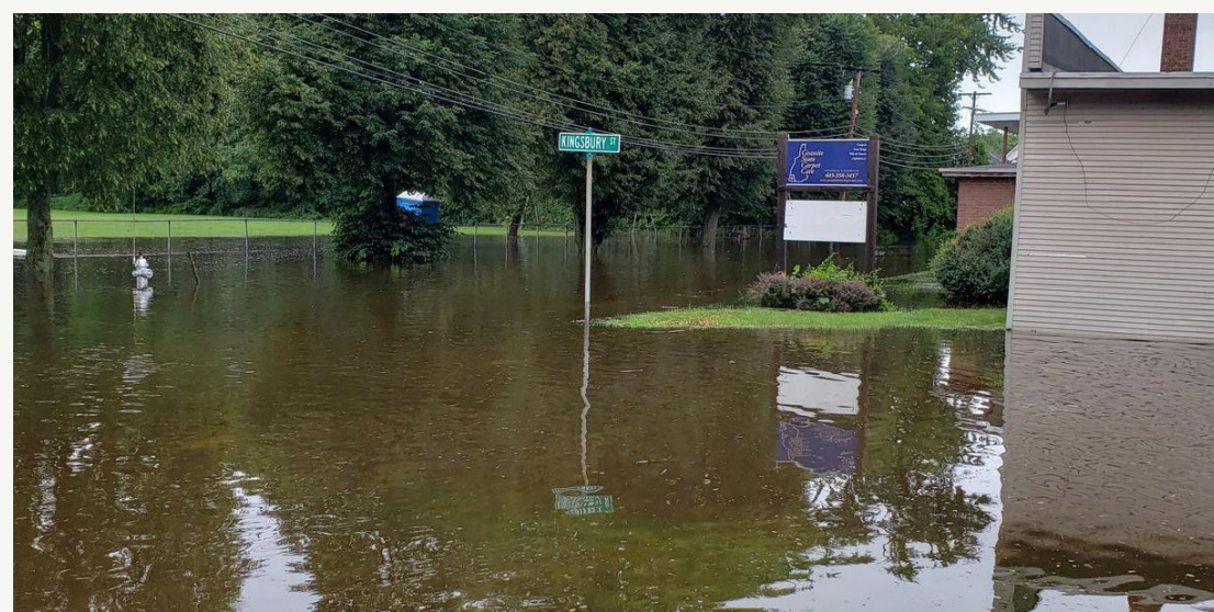
An undersized stormwater collection system along Carpenter Street resulted in frequent flooding of portions of the park and direct discharge of untreated water directly into Beaver Brook.
